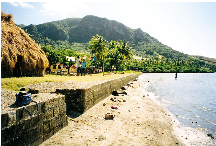
Fig. 4. Vertical seawall (Viti Levu, Fiji)
