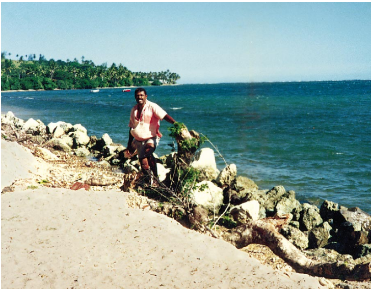
Fig. 3. Coastal protection provided by stones (Viti Levu, Fiji)
