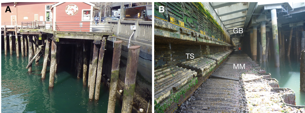
Fig. 1. Seattle seawall, with enhancements, before and after reconstruction. (A) Original seawall. (B) Re-constructed seawall at identical location, shown at an uncommonly low tide. Enhancements for juvenile salmon include marine mattresses (MM) to increase seafloor elevation, a textured seawall and shelves (TS) for invertebrate colonization and fish refuge, and overhanging sidewalk with glass blocks (GB) for increased ambient light
